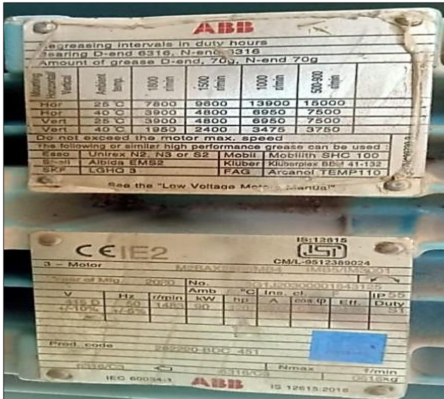
Figure 4: Name Plate Details of 120HP Pump (19)
